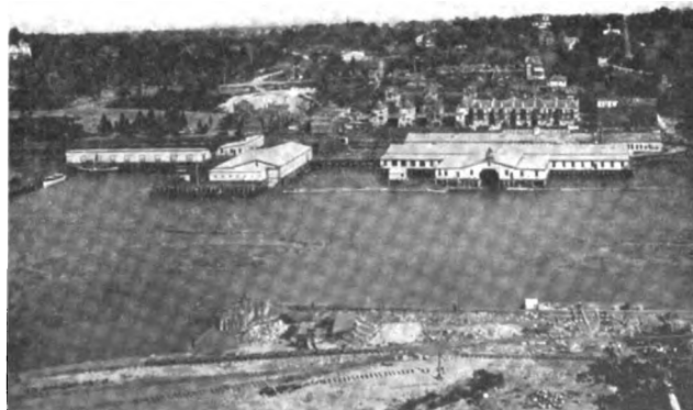
View of the Present Shops
